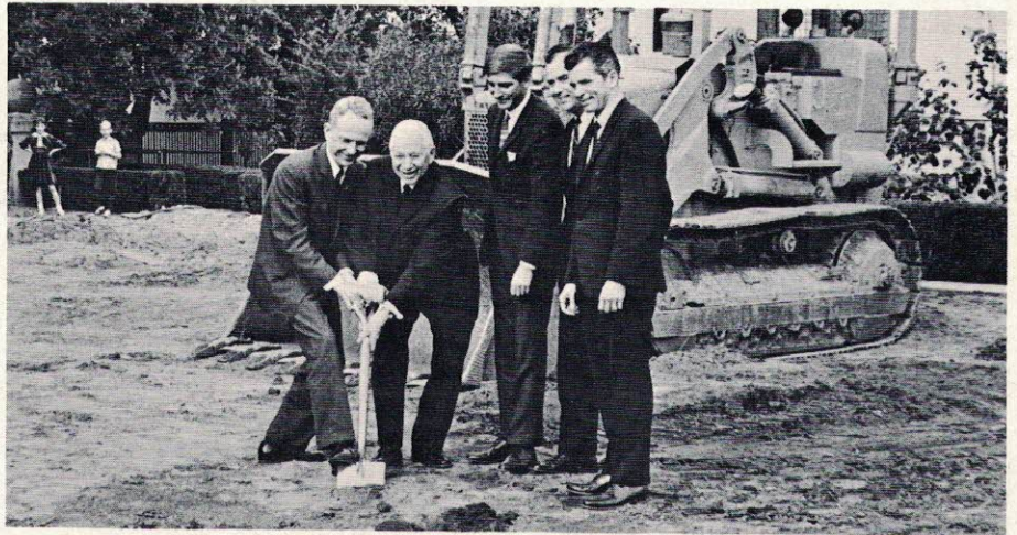
Contractor O. K. Earl assists Mr. Herbert W. Armstrong in breaking the first official ground.
